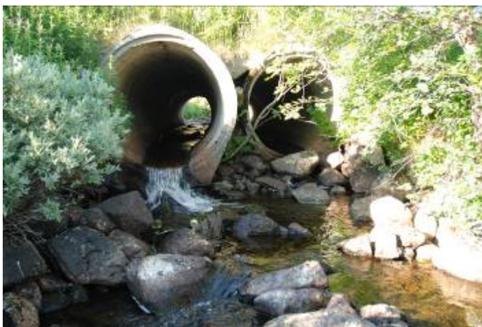
Kulvert under Rv 820
